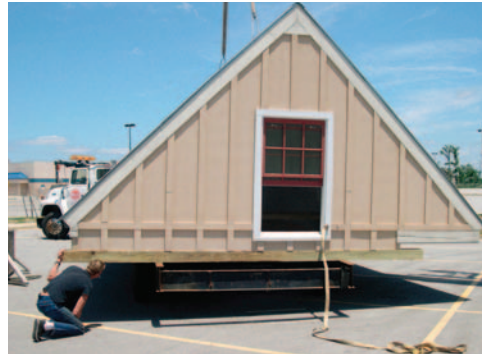
Series of photographs shows roof being lifted off Katrina Cottage with a crane and lowered to the ground; walls are readied for loading for transport. It took only four hours to cut the house apart and prepare it for shipping
