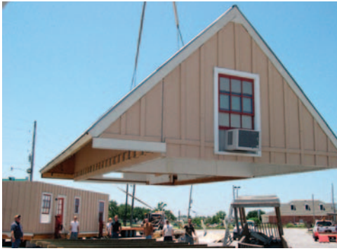
Series of photographs shows roof being lifted off Katrina Cottage with a crane and lowered to the ground; walls are readied for loading for transport. It took only four hours to cut the house apart and prepare it for shipping
