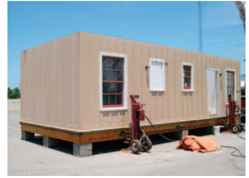
Series of photographs shows roof being lifted off Katrina Cottage with a crane and lowered to the ground; walls are readied for loading for transport. It took only four hours to cut the house apart and prepare it for shipping
