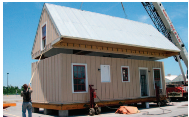
Crew from New Panel Homes, Inc., begins lifting roof.
